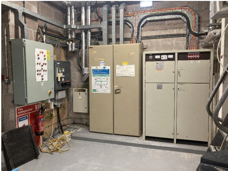
Electricity Supply – Main distribution Board
