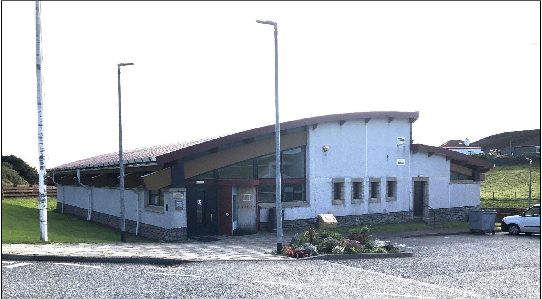
Scalloway Pool Building - Exterior
