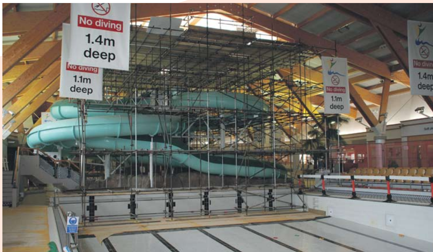
The complex scaffolding structure erected during the pool closure to gain access to repair the roof.
