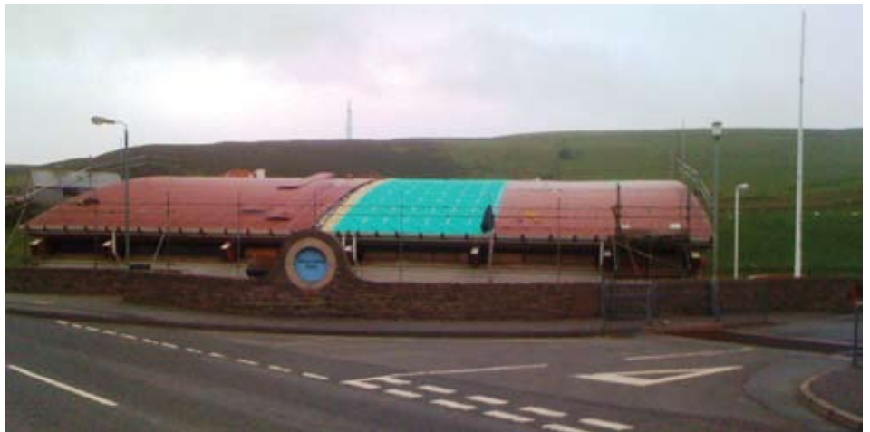
The Scalloway Pool midway through its essential roof replacement during 2012.
